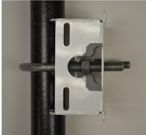
3. Place the angle adapter bracket section on the U-bolt with the open slot connections on the bottom and align it with the pole mount section. Attach with two 1/2 inch nuts. Tighten all nuts to 300 inch pounds (lbf-in).
